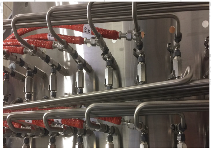
H-Valve panel to supply two robots from a single paint station drop, bulkhead plate mounted and delivered as a single module for installation
